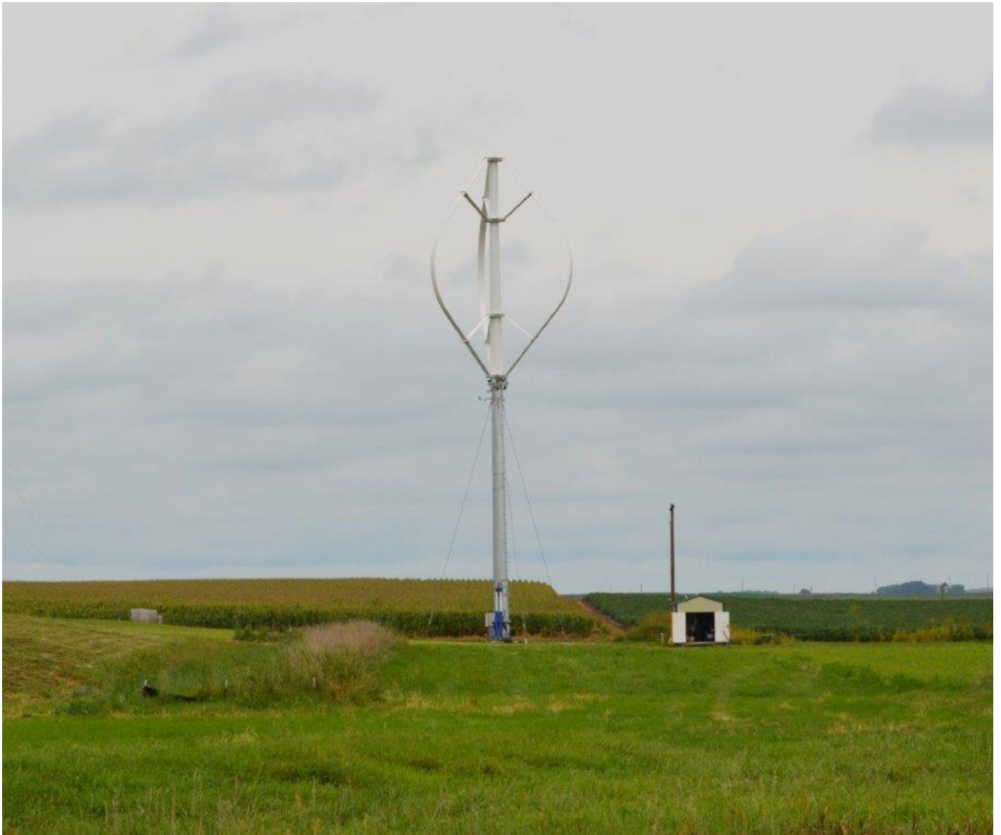
25 KW Chava Wind vertical axis prototype to be used for training and energy for the farm (Pillars 1 and 3).
